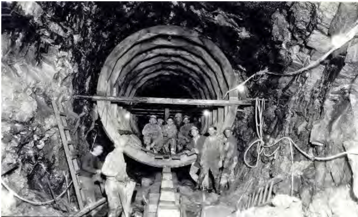
Photo 6. Builders of Quabbin Aqueduct in the Aqueduct
