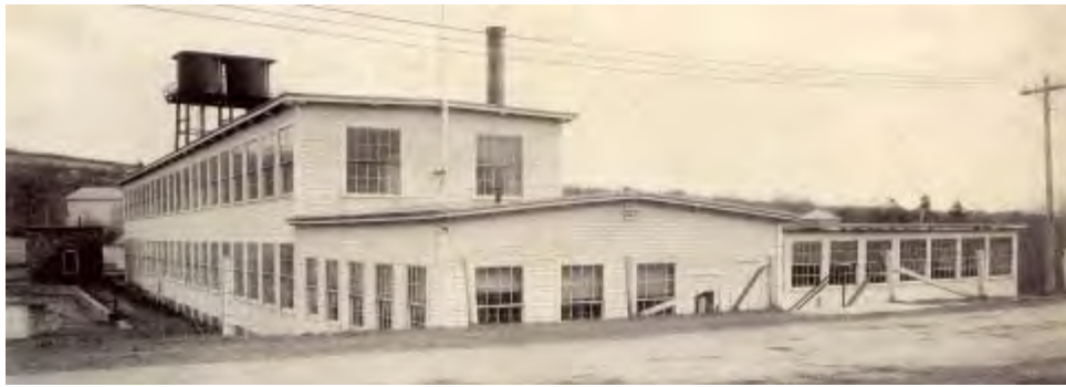
Photo 4. Rutland Worsted Company, West Rutland
